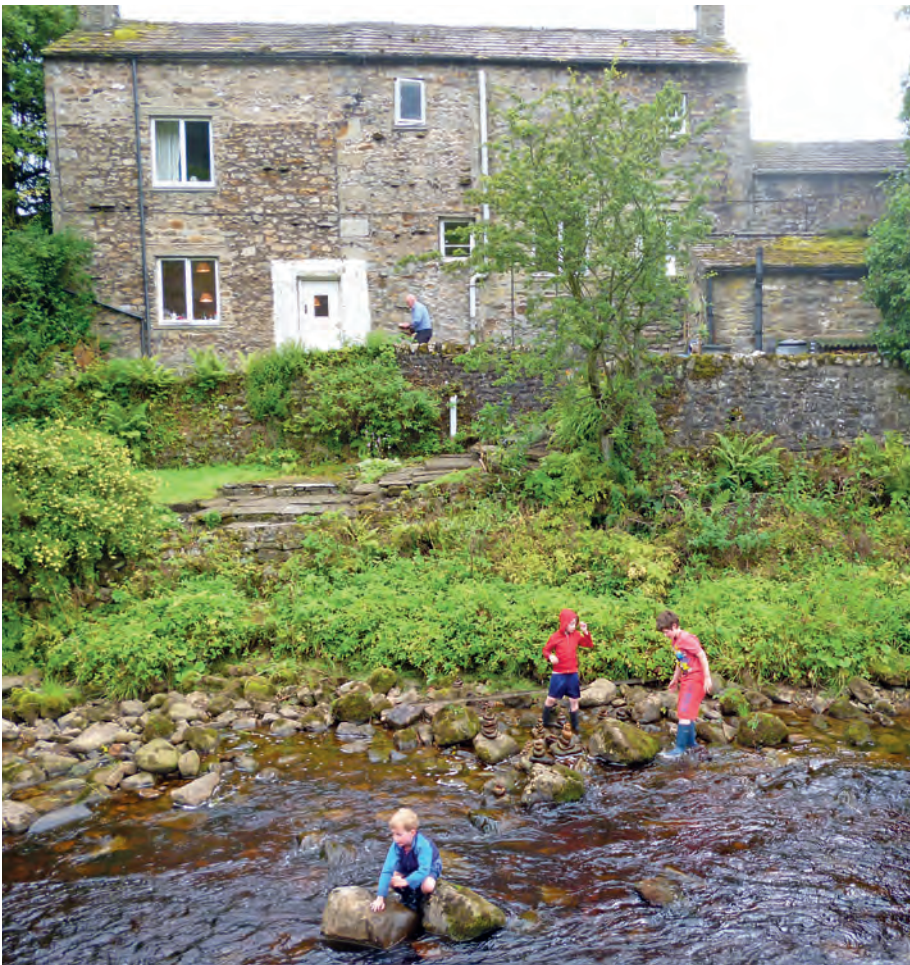
The Bungalow, back view.
